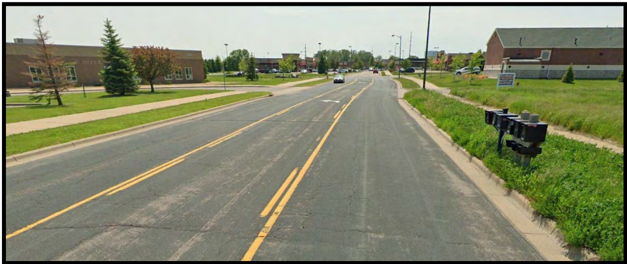
Photo 3. 175 th Street West looking southwest towards Glasgow Avenue.
