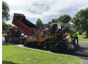
Installation of new asphalt surface
